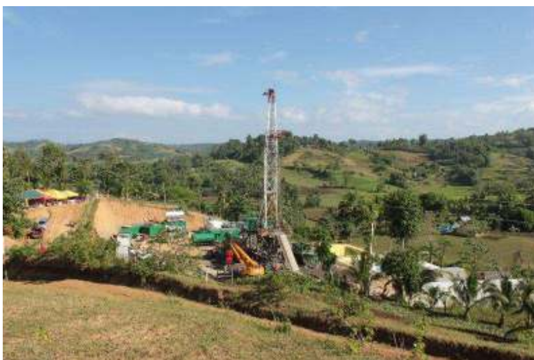
SC 51 Drilling of Duhat-2 well at San Isidro, Leyte
